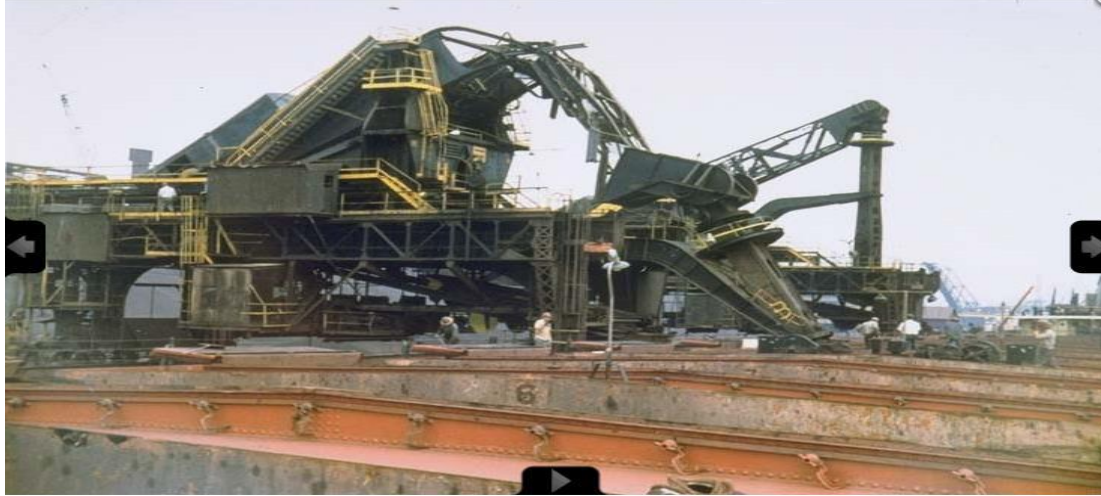
Figure 1-1: Structure failed due to fatigue
